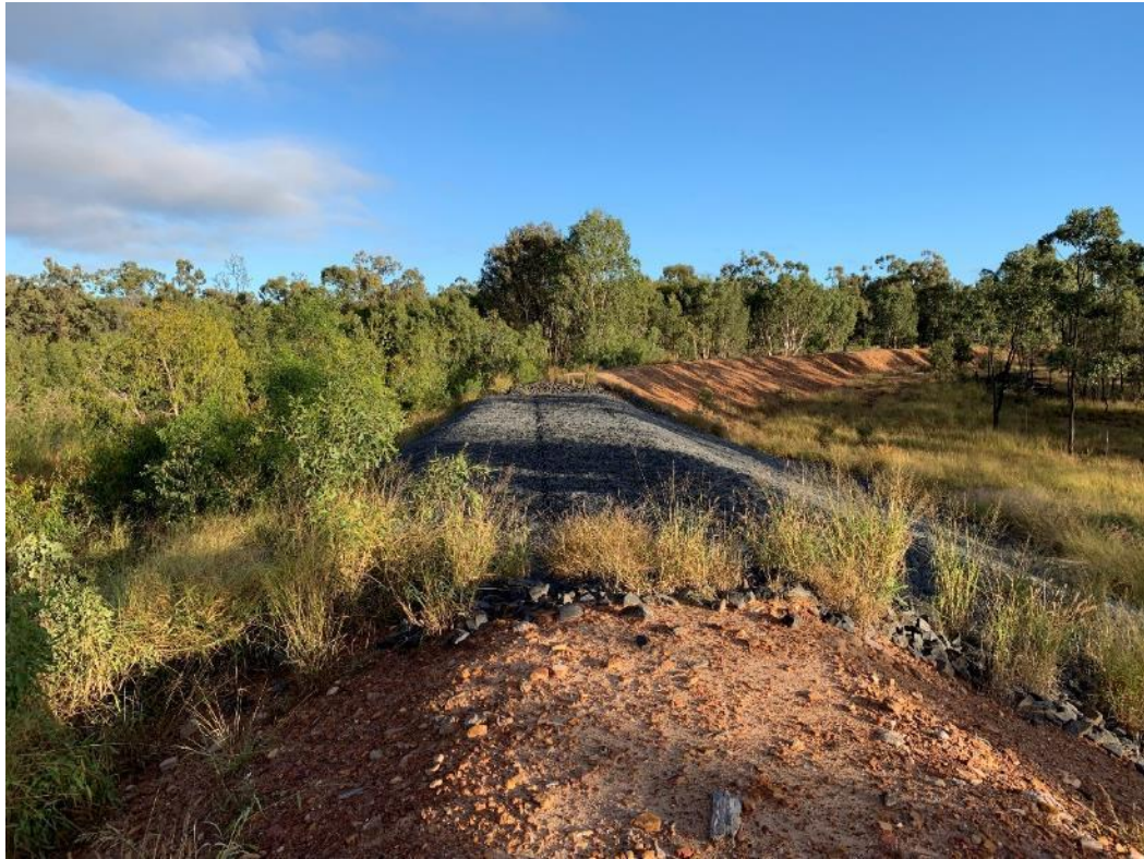
Figure 4.6 - Photograph of the existing drainage diversion and levee within the Project area
