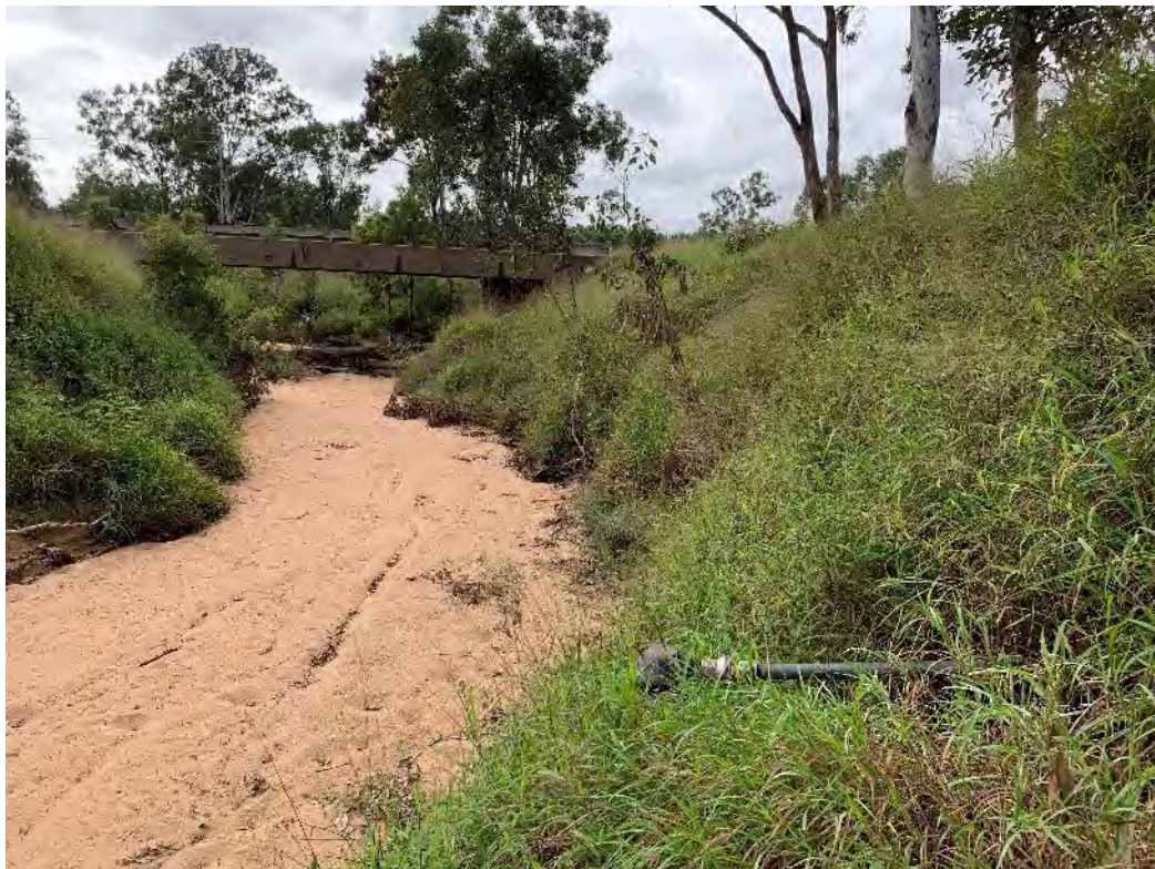
Figure 4.10 - Photograph of Hughes Creek passing under Saraji Road
