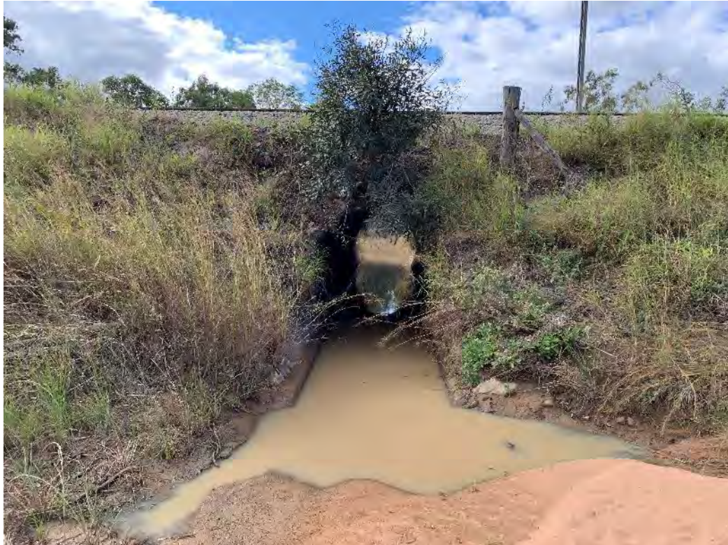
Figure 4.7 - Photograph of Drainage line 6 passing under the Norwich Park Branch railway
