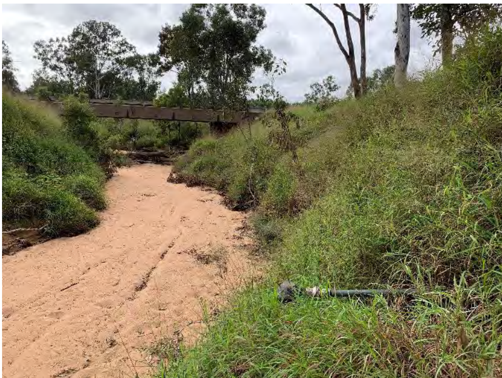
Figure 3.4 Photograph of Hughes Creek passing under Saraji Road
