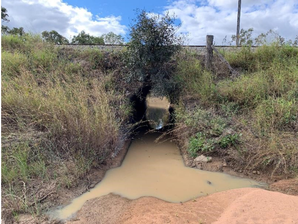
Figure 2.7 Photograph of Drainage line 6 passing under the Norwich Park Branch railway
