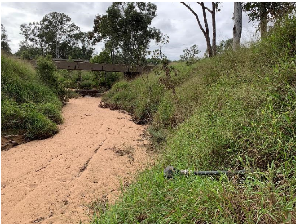
Figure 2.10 Photograph of Hughes Creek passing under Saraji Road
