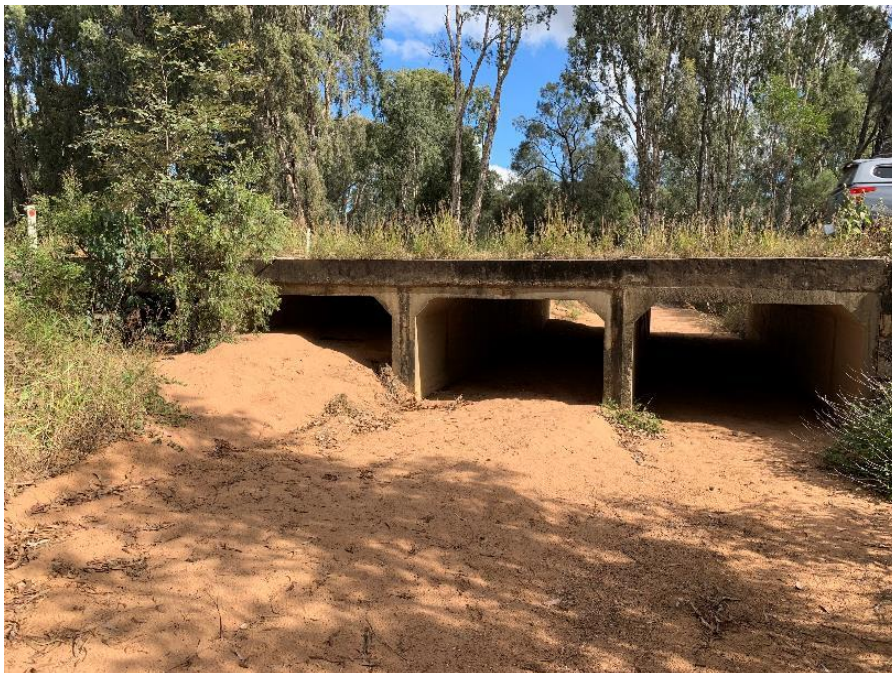
Figure 3.3 Photograph of Drainage line 7 passing through box culverts under Saraji Road
