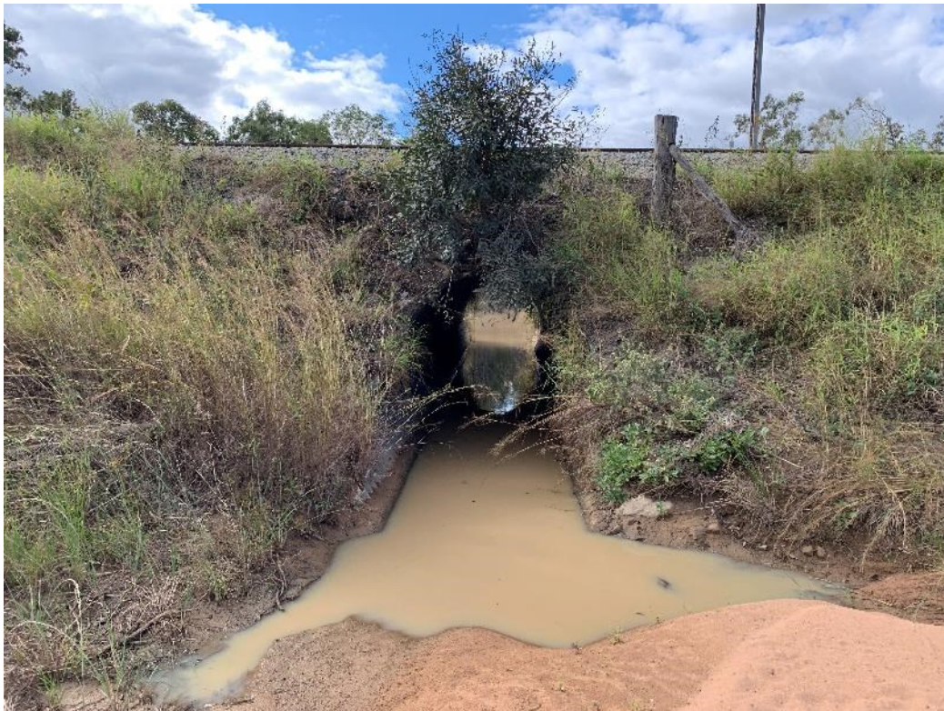
Figure 3.1 Photograph of Drainage line 6 passing under Norwich Park Brach railway
